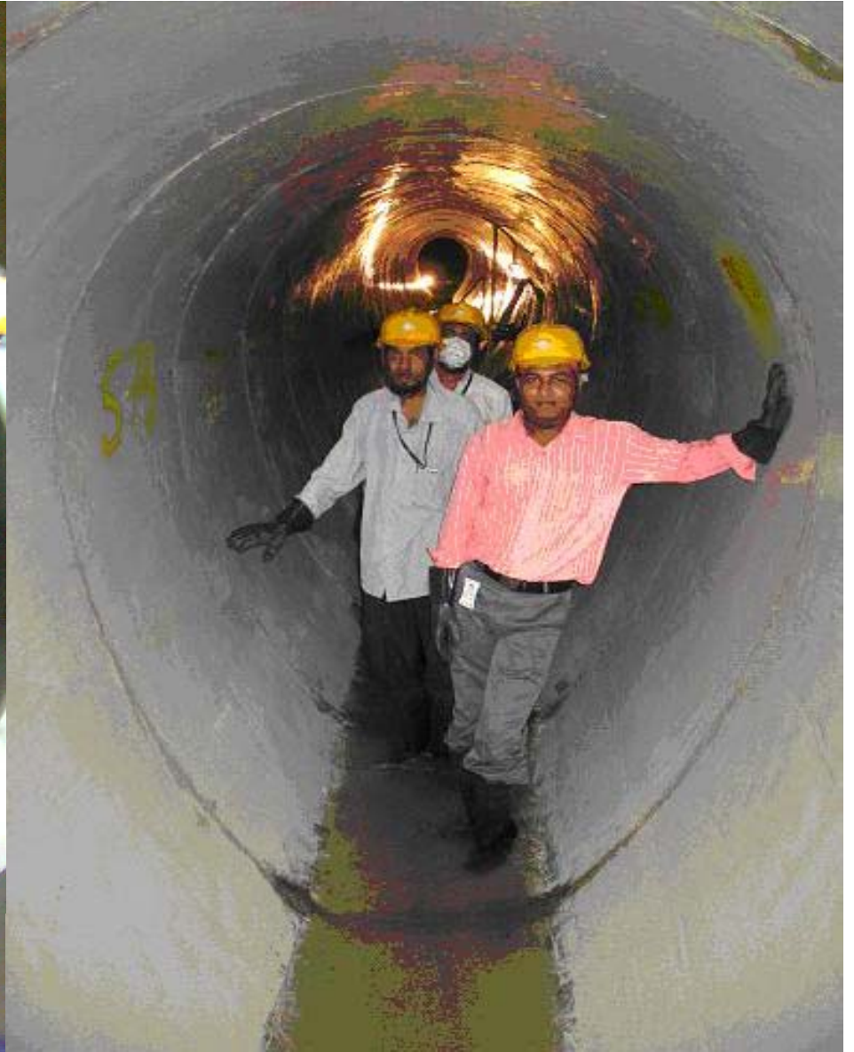
Sewers after lining with GRF lining
